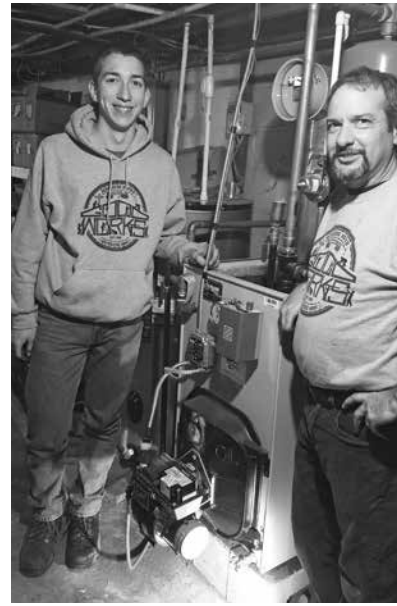
Caleb and Bob working on a furnace
