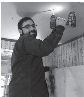
Good Works volunteer replacing water-damaged drywall
