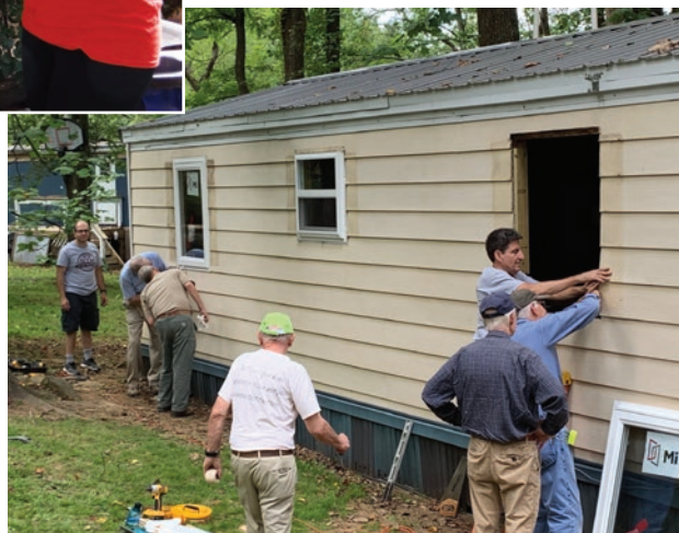
Garden Spot Village volunteers install replacement windows.
